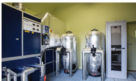
Futuristic plantroom Heavy insulation of all pipes, pumps and filters retains heat
