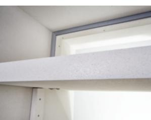
The TROX EK-EU smoke control damper meets the highest test requirements of the EN 1366-10 test standard and is hence unique in Europe.
