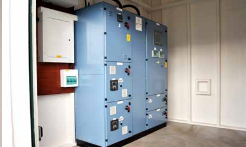
A packaged dosing system from the Verder UK Project Team ready for shipping. The kiosk features a dosing cabinet, chemical storage, control panel, filling ports and booster set
