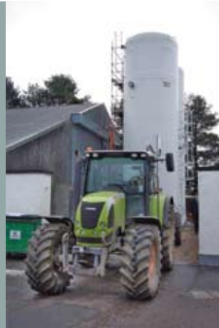
Figure 2 Sludge removal from the bioreactors
