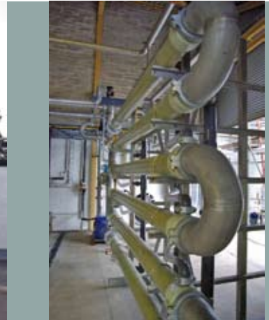
Figure 3 Six ultrafiltration membrane vessels in series
