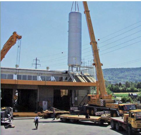
Figure 2 Installation of Wehrle MBR system
