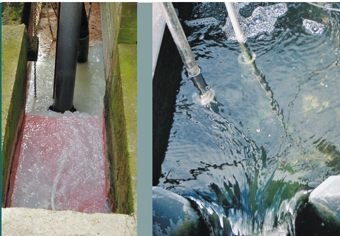
Figure 1 Creamery waste at Inlet to treatment plant and treated effluent prior to river discharge
