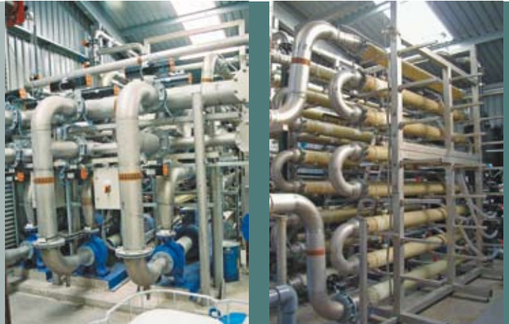
Figure 4 Wehrle UF membrane system
