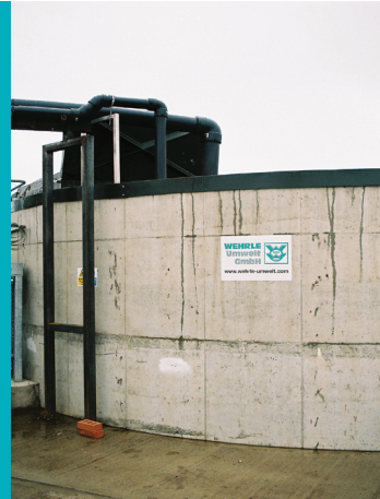
Figure 4 Biological Treatment Tank
