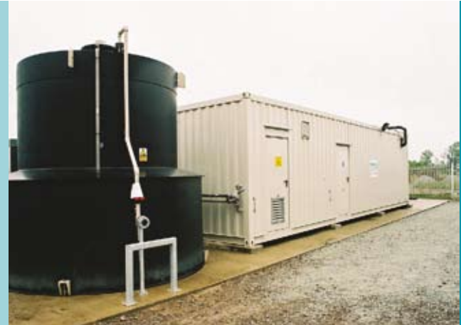
Figure 2 Containerised Wehrle membrane system
