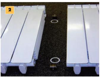
Screw a pair of nipples into one end of the radiator.
