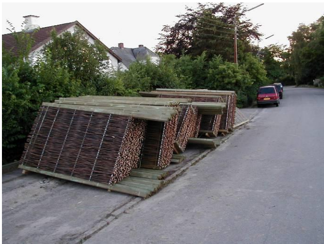
Dried willow panels delivered and ready for installation.
