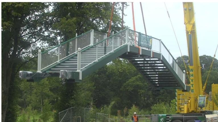
The main central span was lifted onto the two stone piers using a 350t crane. The two side spans were then placed and site welded into position.
