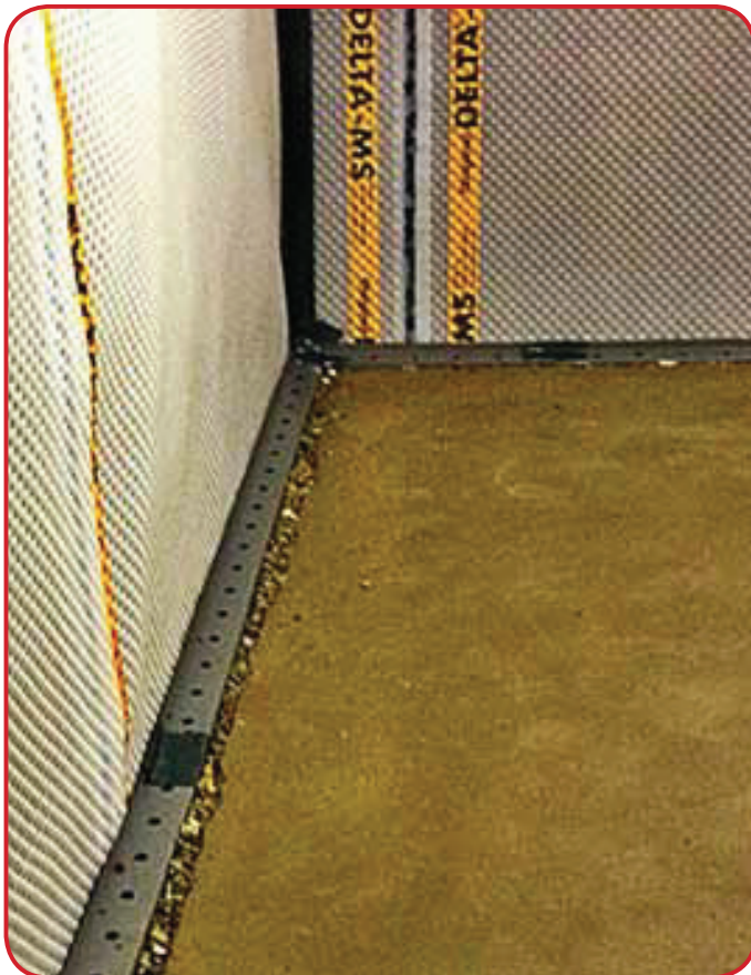
Typical 'Perimeter Channel' installation
