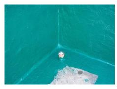
liquid applied gas membrane. It offers a simple, continuous passive gas prevention barrier against the ingress of Methane, Carbon Dioxide, Radon, Ground Gas, VOC, air & Moisture into buildings. **LGB** also acts as a waterproofing membrane complying with C2 and C4 schedule 1 of the Building Regulations 1991 for England and Wales. MemTech LGB meets the requirements of BS8485:2015.
