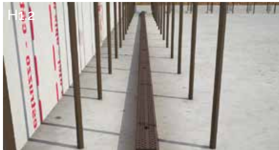
H1.1/H1.2 HORIZONTAL CONSTRUCTION JOINT (COLD JOINT) - RAFT FOUNDATION WITH DELTA AMPHIBIA
