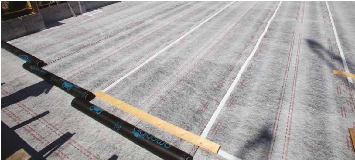
RAFT FOUNDATION WITH DELTA AMPHIBIA SYSTEM
