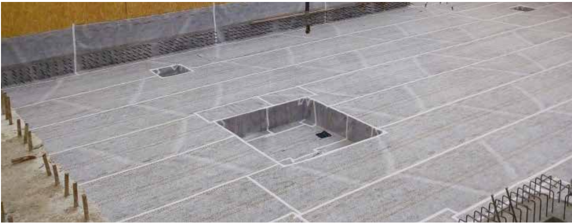
LIFT PIT WITH DELTA AMPHIBIA SYSTEM
