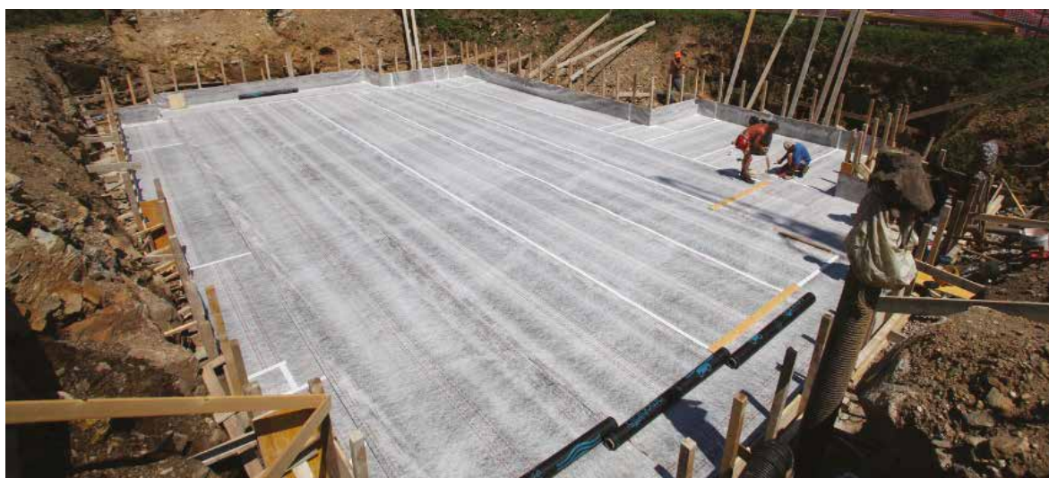
RAFT FOUNDATION WITH DELTA AMPHIBIA SYSTEM
