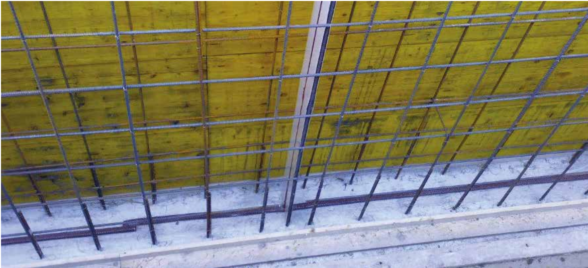
APPLICATION OF SELF-SEALING STRUCTURAL CRACK INDUCER BREAK
