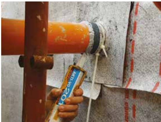
02.1/02.2 | DELTA AMPHIBIA INSTALLED ON SLURRY WALLS/EXISTING STRUCTURES- SEALING OF PENETRATIONS
