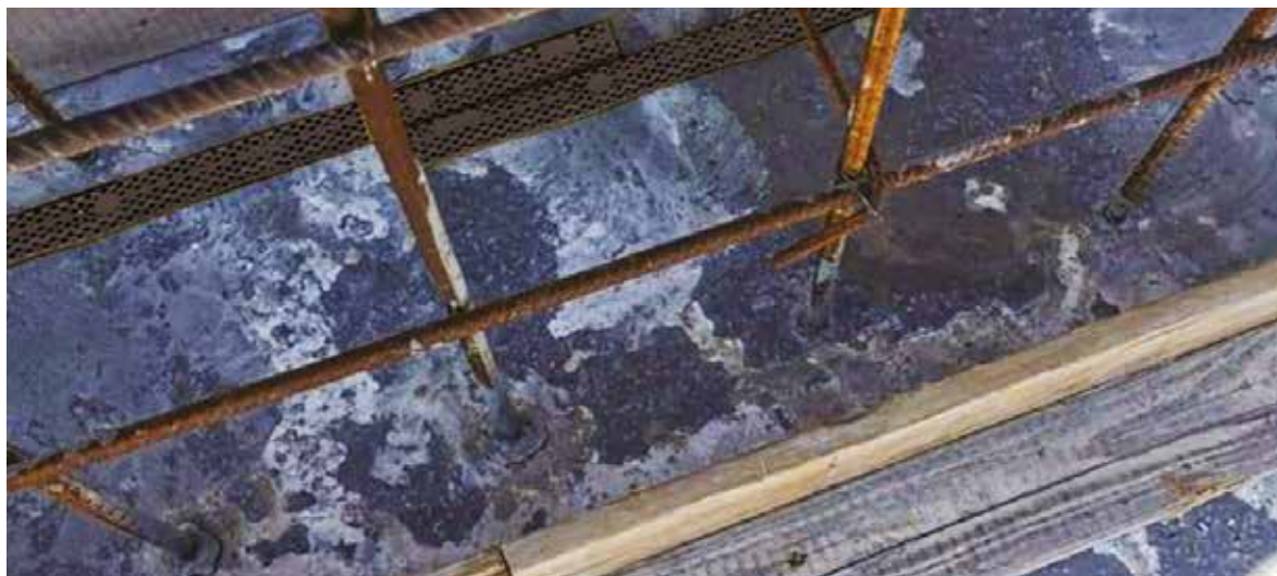
DETAIL OF BENTONITE SWELLABLE KOSTER WATERSTOP KOSTER QUELLBAND
