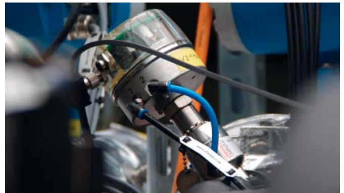
GEMÜ 650 diaphragm valves with combi switchbox GEMÜ 4222
