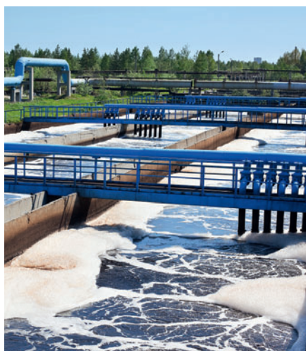
Classic activated sludge basin
