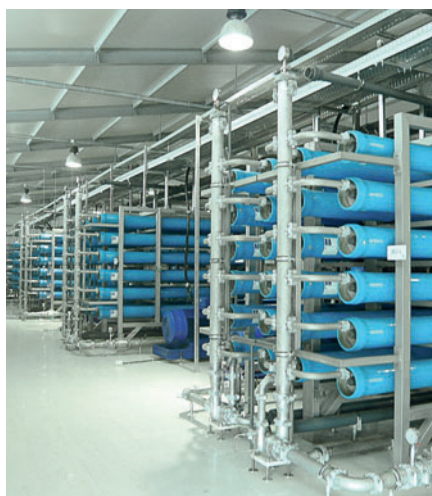
Reverse osmosis system. Source: Watertec T.A. GmbH
