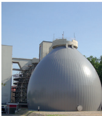
Digester. Source: Dahlem Beratende Ingenieure
