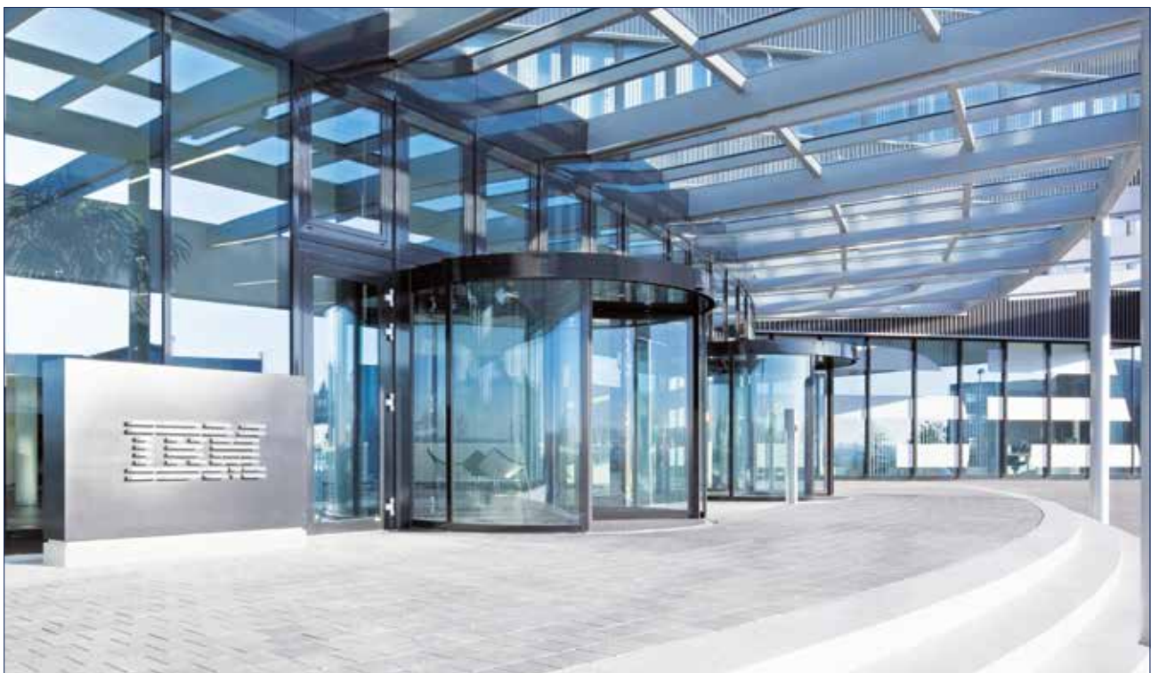
IBM Ehningen, Germany (Photo: GEZE GmbH)
