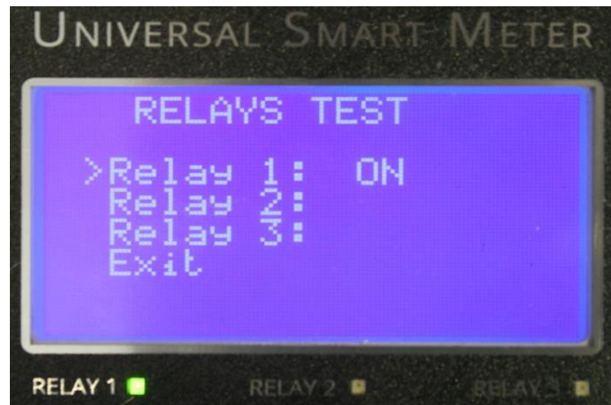
Figure 6.2 – Relays Test Screen 2
