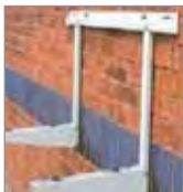
Wall mounted bracket & condensate tray
