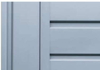
Joint profile between horizontal and vertical cladding
