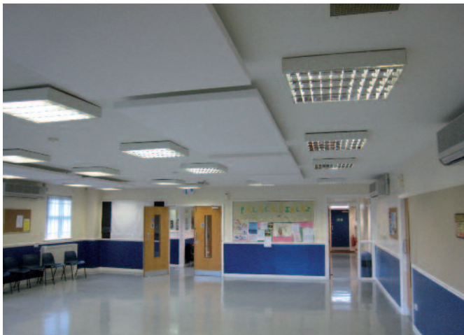
Sonata Vario absorbers fixed to a ceiling.
