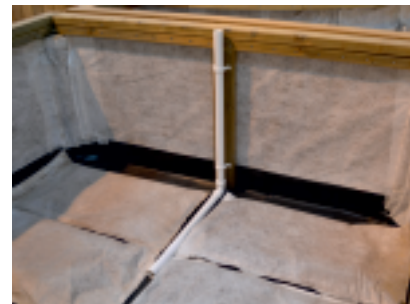
Hydroleca sacks laid out in base of planter
