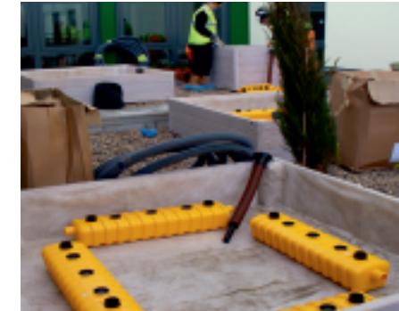
Water storage tanks and filler pipe
