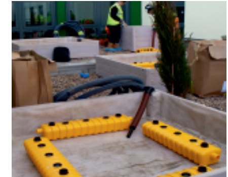
Water storage tanks and filler pipe
