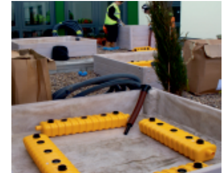
Water storage tanks and filler pipe
