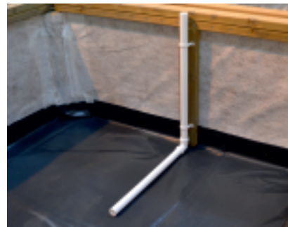
Polythene liner with filler pipe
