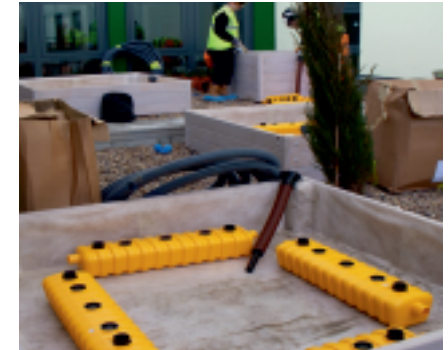
Water storage tanks and filler pipe
