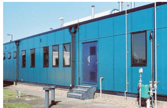
Plastisol steel FR, plywood core, drip rail, parapet capping and powder coated aluminium caps as detail (d), page 11
