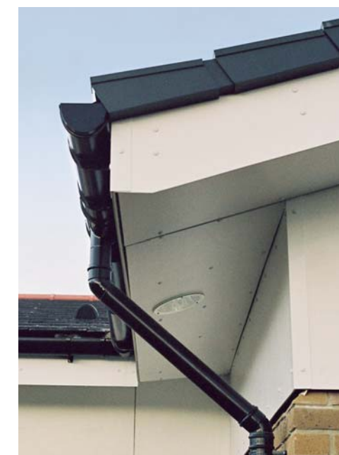
Vulcatuf® screwed to timber frame on soffit, fascia and barge board
