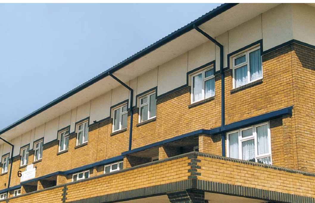
Vulcatuf® riveted to steel lugs as detail (b), page 10
