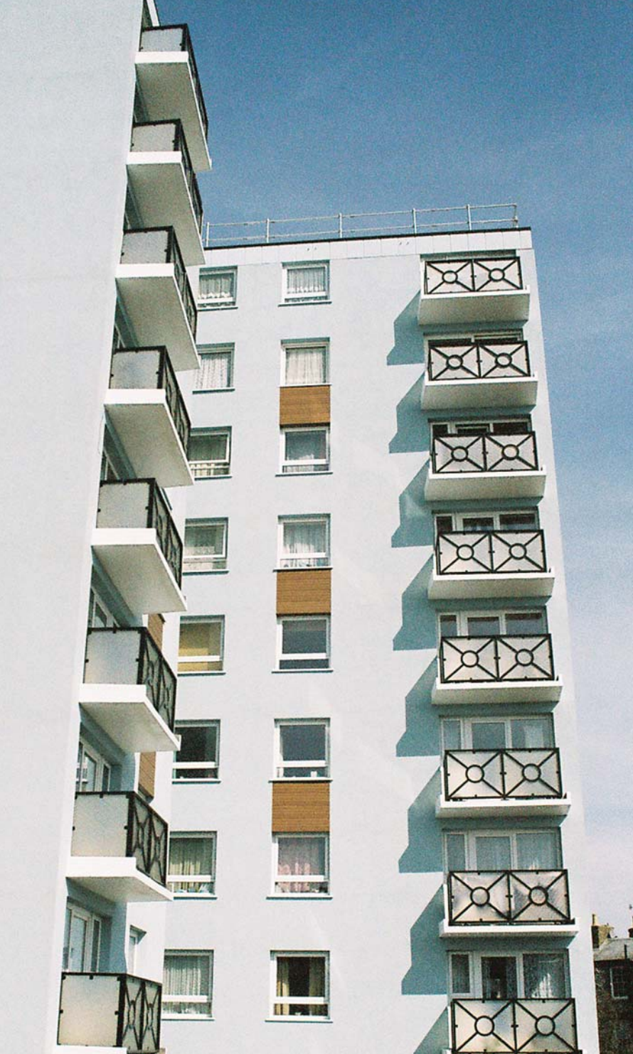
Balcony panels bolted to lugs as detail (b) page 10. Also WeatherTone ® prefinished timber shiplap in walnut.
