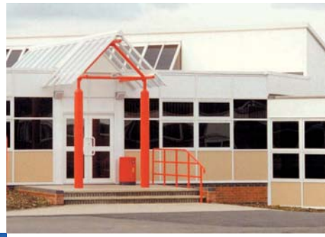
GRP faced 24mm thick infill panels
