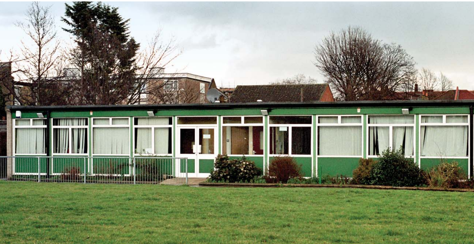
Plastisol steel faced 28mm thick with outside face reinforced with 4mm plywood
