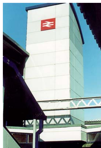
Vulcatuf® riveted to steel lugs as detail (b), page 10
