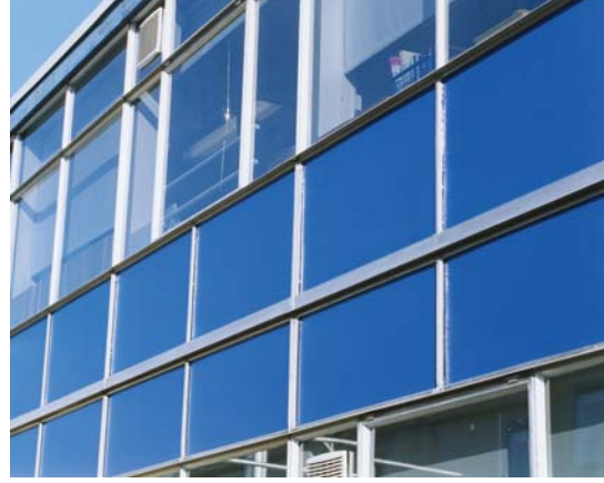
Trespa faced 32mm thick with white plastisol rebated inside face and 16mm thick edges
