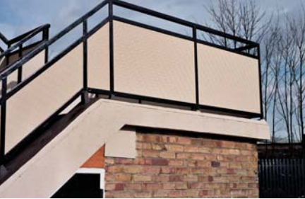
Deep crinkle texture double sided Vulcatuf® fixed with powder coated aluminium black beads, as detail (g), page 11
