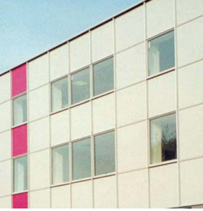
GRP faced 28mm thick infill panels Class 1 FR grade
