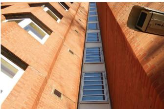
The Em-Louvre is a high-performance smoke vent which draws smoke and toxic fumes from buildings fast. Em-Louvre smoke vents increase occupier and building safety in apartment and commercial buildings – especially high-rise configurations, thanks to superior resistance to weather and wind load. We've designed them for easy, rapid installation into façade apertures and curtain walls.
