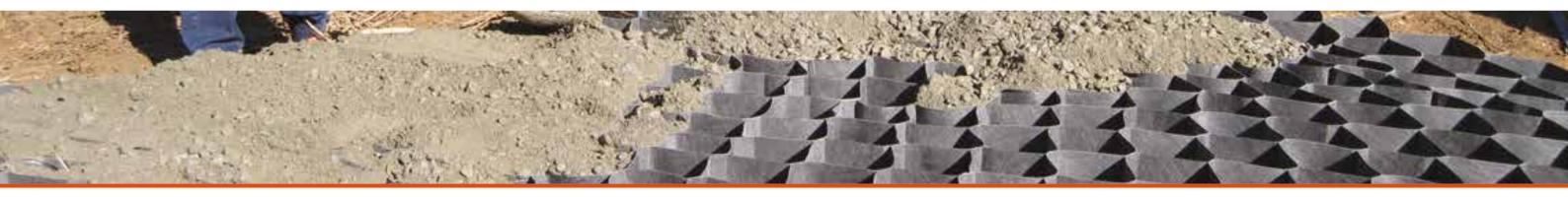
Protect tree roots from vehicle traffic, whilst maintaining water and nutrient absorption using TERRAM GEOCELL.
