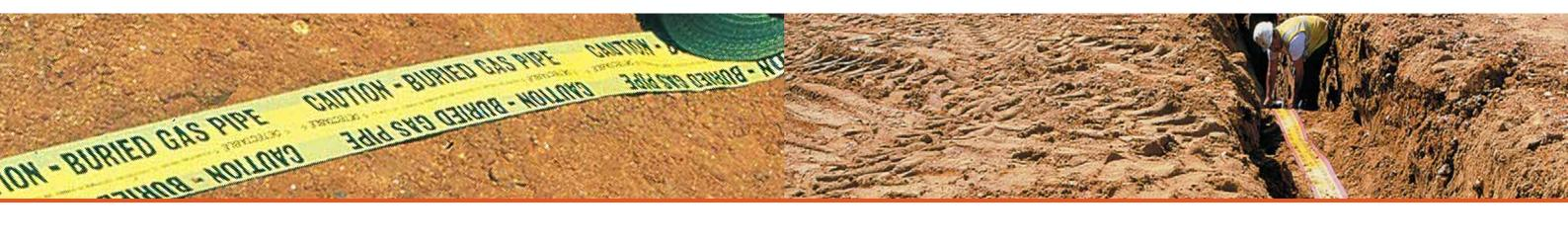
Underground tapes with an aluminium foil tape are used to mark, warn and allow the detection of buried underground pipes and cables.
