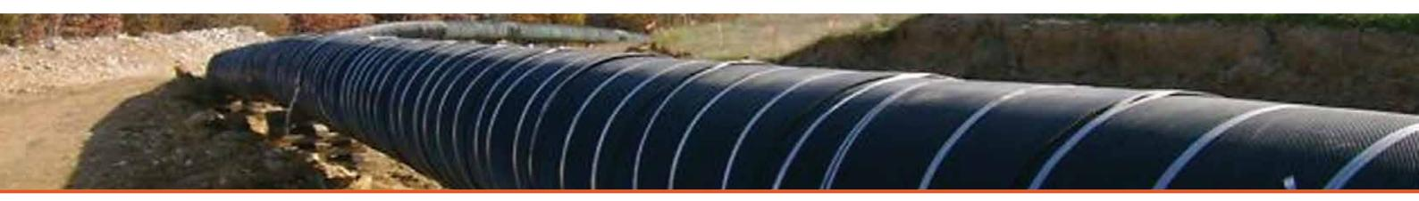
Flexible mesh products are used in major pipeline projects to replace the thick sand collar that would traditionally have been placed to cushion the protective coating around a steel pipe.
