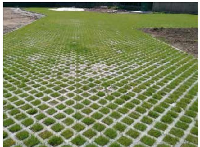
Not only was TERRAM Truckpave easy to install but unlike honey-comb cell type plastic pavers, it resists rotation and displacement caused by heaving vehicle movements.
