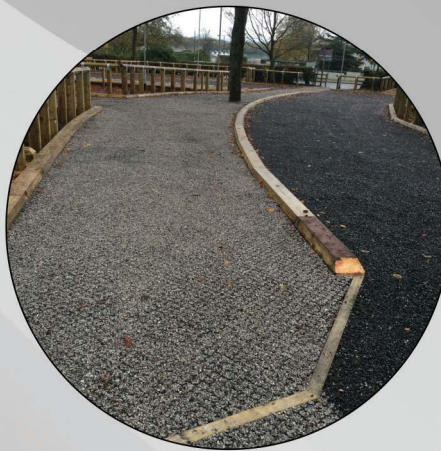
Backfilled with gravel
