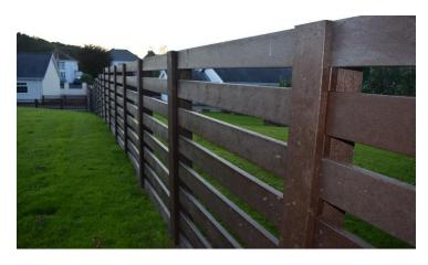
Face boards can also be used to allow the free movement of the boards allowing for the maximum amount of expansion and contraction.
