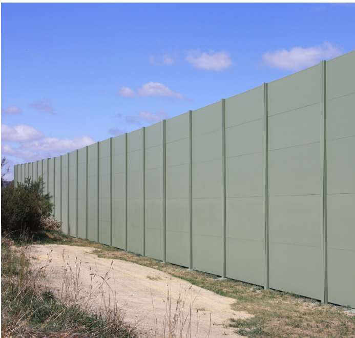
GuardianWall™ - Waste Transfer Station
