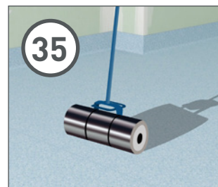
35 Roll with a 68kg articulated floor roller, firstly in the short direction, then in the long. In corners and other awkward areas, use a hand roller. Ensure that all the sheets are adhered.
