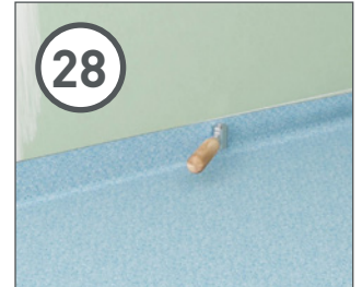
28 Use a hand roller along the wall to firmly press the vinyl into the adhesive and create a strong bond.
