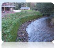
Flex MSE's® engineered geomodular system was chosen as a flexible, simple to install solution that would provide high & low-level protection against scour, erosion & flood events.
