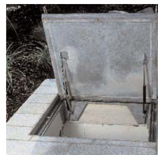
HINGED PAN COVER WITH LIFT ASSIST
