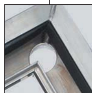
Top-side - Water drainage channel with drainage outlet
