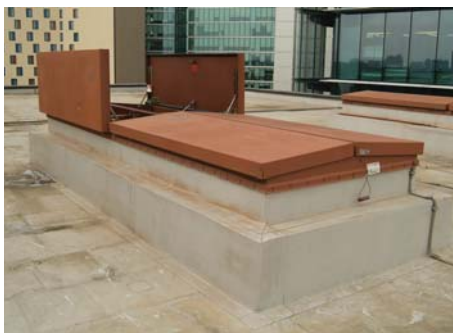
Type ACDSH acoustic smoke vents.
