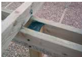
....joint fixed over the beams....
