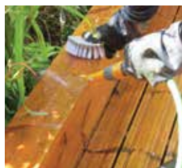
Q-Deck® Lunawood being cleaned with Net-Trol.
