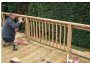
....fixing the balustrades....
