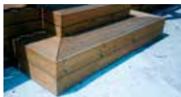
Steps can be created by extending different levels of sub frame.
