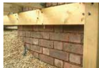
....ledger board fixed to existing wall....
