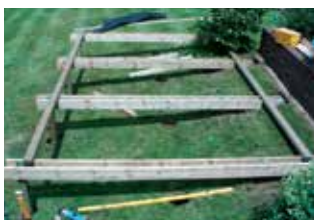
....building the support beams....
