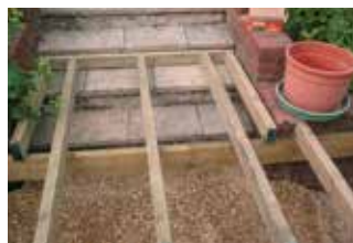
....ledger board fixed to existing steps....
