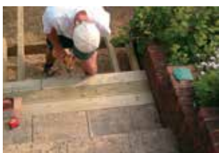
....fixing the first deckboards....
