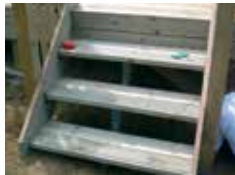
Step frame set on compacted hardcore and weed barrier.
