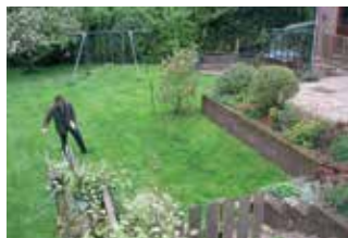
Checking the deck location....
