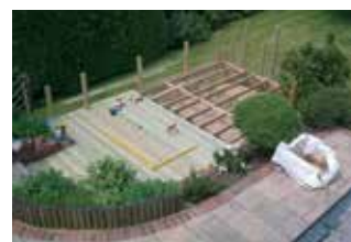
....fixing the deckboards throughout the deck....
