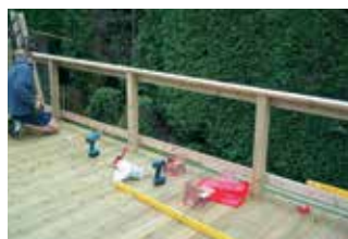
....fixing the handrails and base rails....
