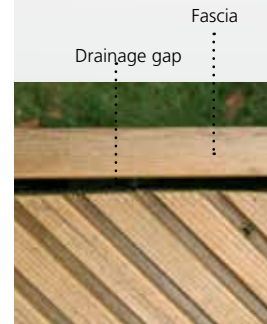
Fig (i) Boards placed at right angles to pedestrian traffic.
