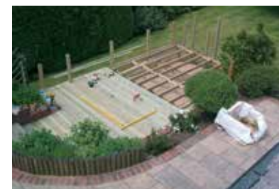
....fixing the decking boards throughout the deck....
