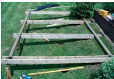
....building the support beams....
