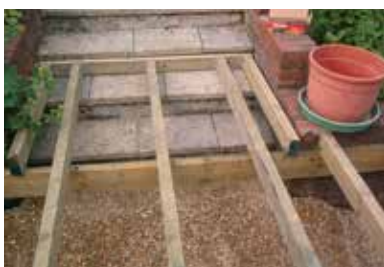
....ledger board fixed to existing steps....
