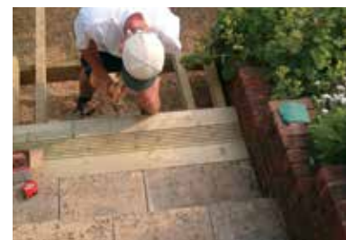
....fixing the first decking boards....
