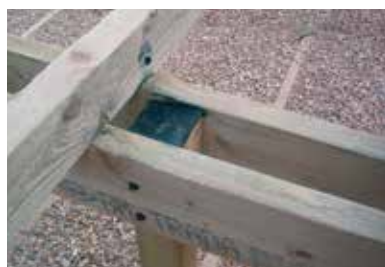
....joist fixed over the beams....
