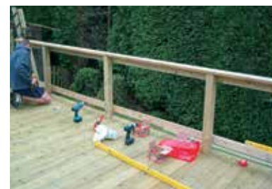
....fixing the handrails and base rails....
