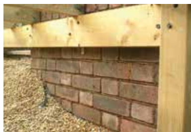
....ledger board fixed to existing wall....
