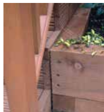
Timber-Tite countersunk versus proud hex head.
