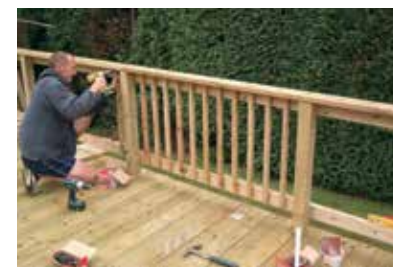
....fixing the balustrades....
