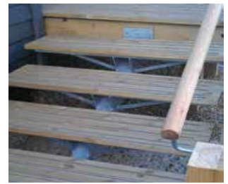
Q-Grip Strips fitted into Q-Deck
