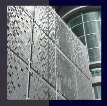
The STEREO-KINETIC® façade was mounted on an independent steel frame which was bolted back to the existing structural steelwork.
