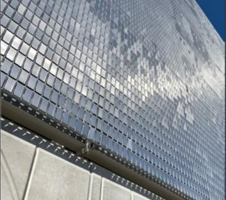
Lang+Fulton work closely with the architect from concept to final design, preparing CAD drawings and advising on support steelwork, alternative fixing methods and loading specifications to current British Standards.
