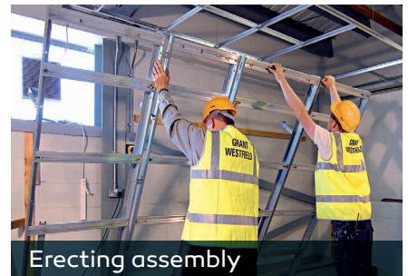
Assembling module frames
