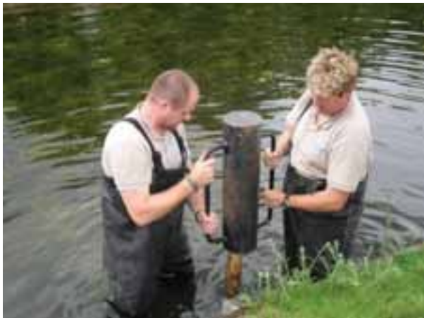
Hampton Court staff installing coir rolls
