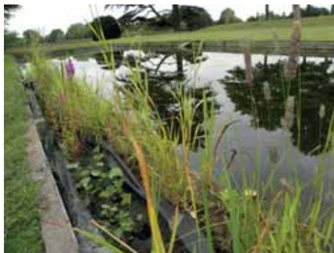
Finished backfill planting behind coir rolls at Klon Dyke
