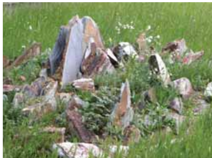
Rockery on biodiverse greenroof to provide solution for extreme wind scouring of substrate, which was preventing vegetation establishment
