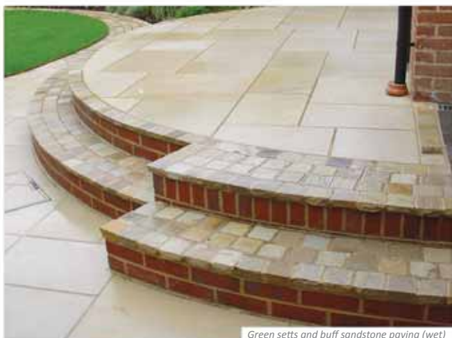
Green setts and buff sandstone paving (wet)
