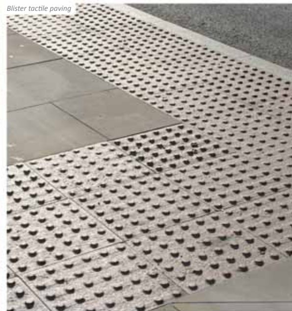
Blister tactile paving
