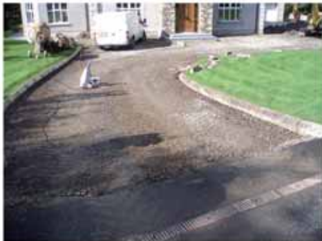
4.) Place the sheets over the prepared ground
