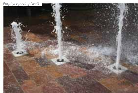
Porphyry paving (wet)
