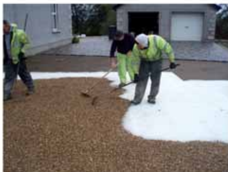
5.) Fill the sheets with gravel
