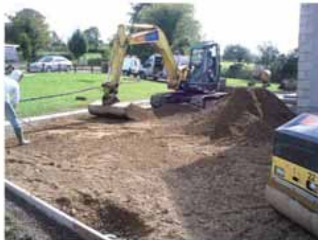
5.) Fill the sheets with gravel
