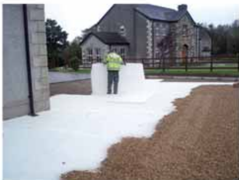
4.) Place the sheets over the prepared ground
