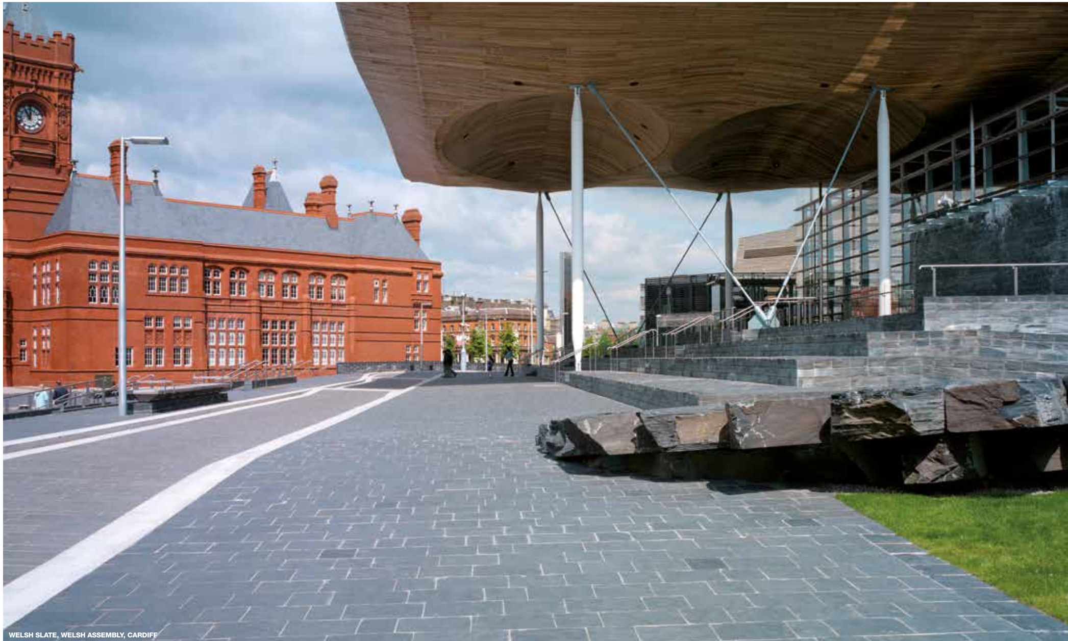
WELSH SLATE, WELSH ASSEMBLY, CARDIFF
