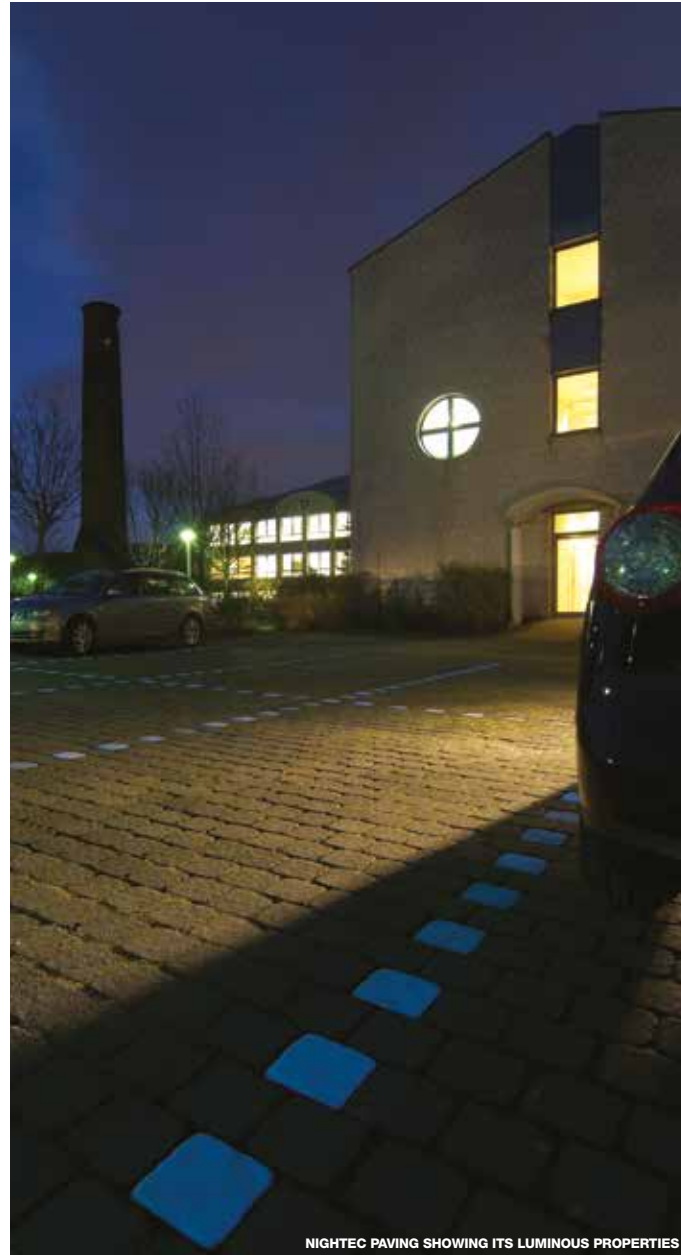
NIGHTTEC PAVING SHOWING ITS LUMINOUS PROPERTIES
