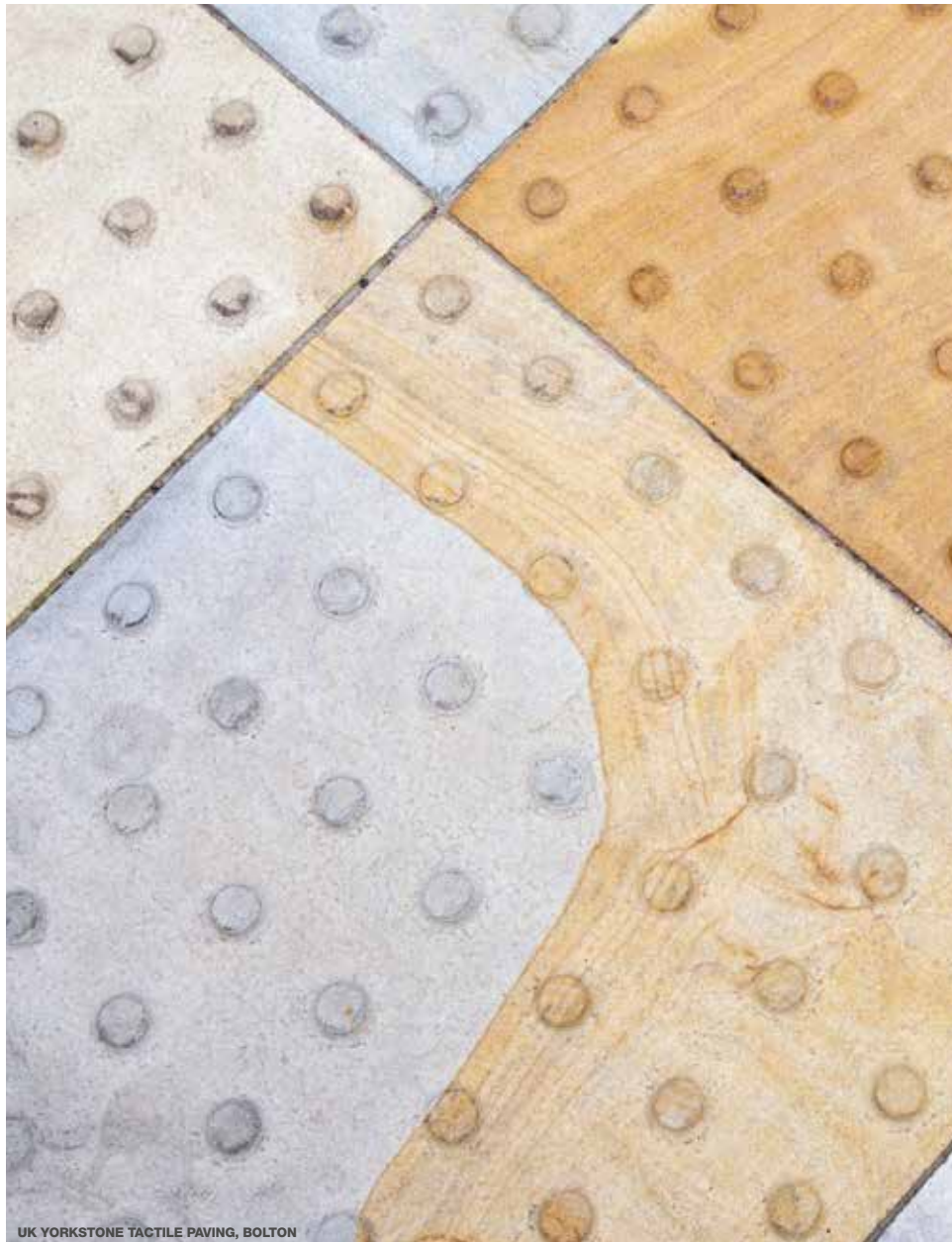
UK YORKSTONE TACTILE PAVING, BOLTON
