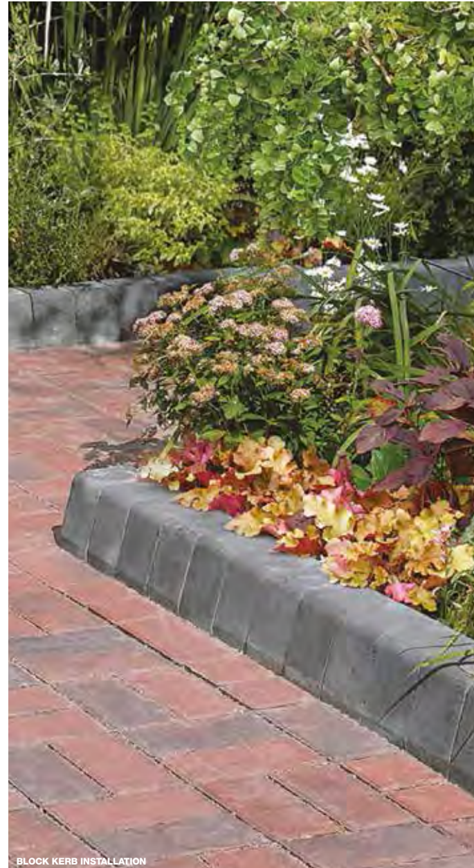
BLOCK KERB INSTALLATION
