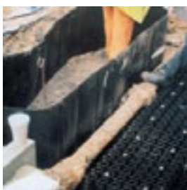
ReRoot 1000 installed to protect underground services and divert roots beneath pavement surfaces
