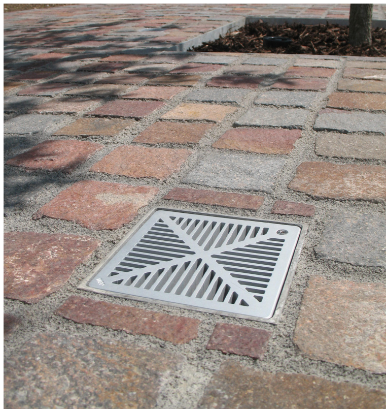
The Arborvent is frequently used to provide several irrigation/aeration points around individual large trees in conjunction with the RootCell system.
