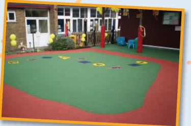
• **THE THICKNESS OF WET POUR RUBBER** laid is dependent on the critical fall height required, if existing play equipment is present, and by the base onto which the surface is being laid. The base can consist of an existing well drained hard surface, newly installed tarmacadam or concrete, or compacted crushed stone such as type 1 MOT.
