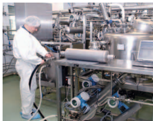
Calibrating flowmeters on-site with the mobile calibration rig
