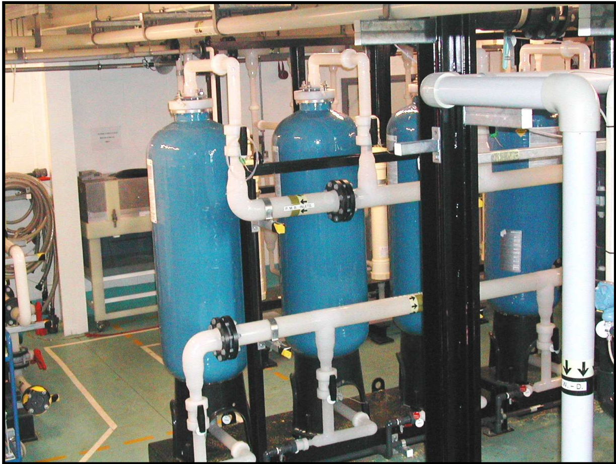
High Purity Ion Exchange Polishers
