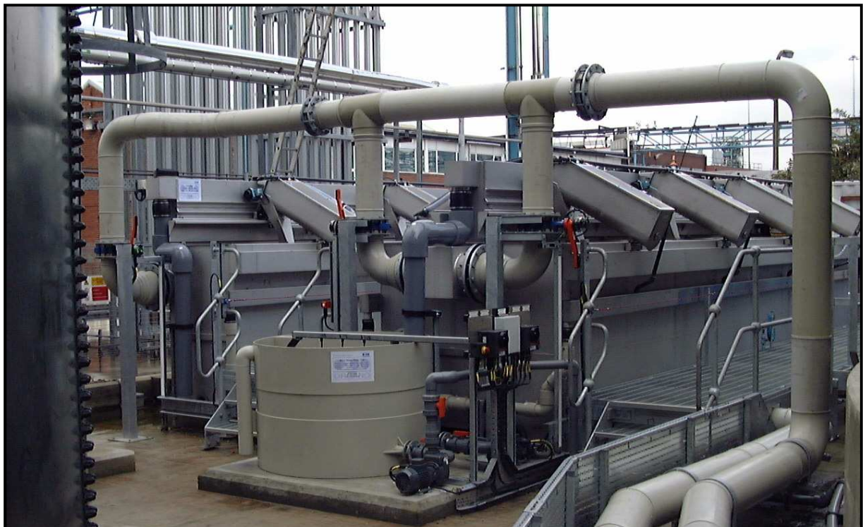
End view of the two filters showing the wash water supply system in the foreground
